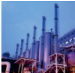
Category C3/C4 chemical industries
